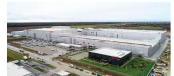
Project Name : SKBH 1st & 2nd Hook-Up Construction Client : SK Innovation (Komarom, Hungary) PJT Period : 2019~2020
