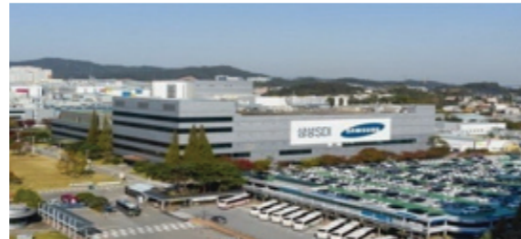
Project Name : SDI Cheon-An M2 Facility Hook-up Construction Client : Samsung SDI (Cheon-An) PJT Period : 2023
