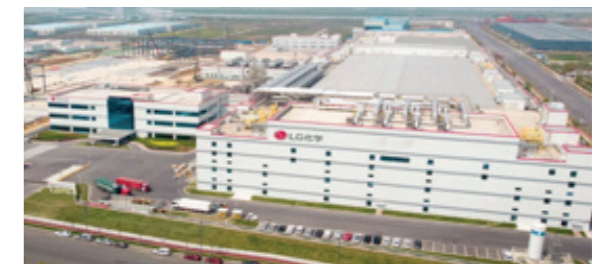
Project Name : LGCNB Coater Heat Exhaust Duct & Hot Oil Pipe Construction Client : LG Energy Solution (Nanjing, China) PJT Period : 2019
