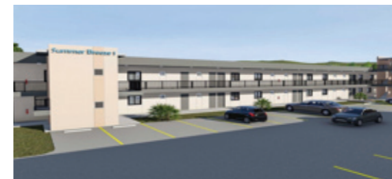
Project Name : Summer Breeze, Vista Facility Construction Client : Core-Tech (Guam, U.S.) PJT Period : 2022~Processing
