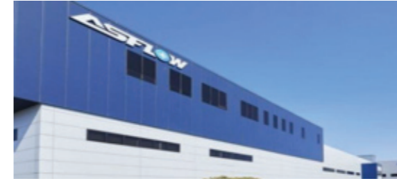
Project Name : Asflow #1,2 F/L ICR Construction Client : Asflow (Hwa-Seong) PJT Period : 2019~Processing
