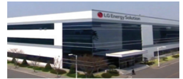
Project Name : LG Energy Plant HVAC Steam-coil Replacement Client : LG Energy Solution PJT Period : 2023
