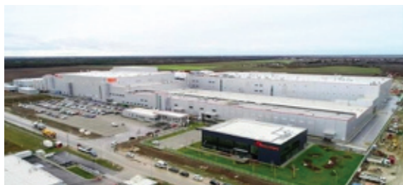
Project Name : SKBH Dry Room Construction Client : SKInnovation (Komarom, Hungary) PJT Period : 2018~2020
