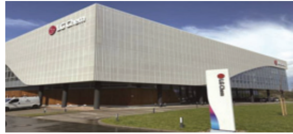
Project Name : LGCHEM DR HVAC Construction Client : LG CHEM (Cheong-Ju, O-Chang) PJT Period : 2010~Processing
