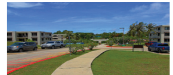
Project Name : P309 Navy Combat Element Construction Client : GO JV(Guam, U.S.) PJT Period : 2023~Processing
