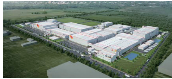
Project Name : SKIHU Battery 1st Factory DR Design Engineering Client : SK Innovation (Komarom, Hungary) PJT Period : 2017~2018
