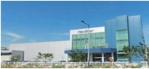
Project Name : CLEAN ROOM SYSTEM Construction Client : Nextstar Energy (Hwa-Seong) PJT Period : 2012 ~ 2020
