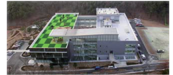
Project Name : Yong-In R&D Center Clean Room Construction Client : Samsung Tales (Yong-In) PJT Period : 2014
