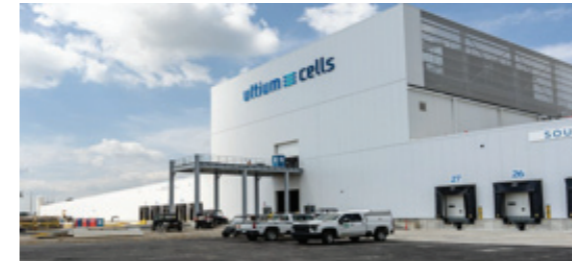
Project Name : Electrode Coater Heat Exhaust Duct & Hot Oil Pipe Construction Client : Ultium Cells(Ohio, U.S.) PJT Period : 2021~Processing
