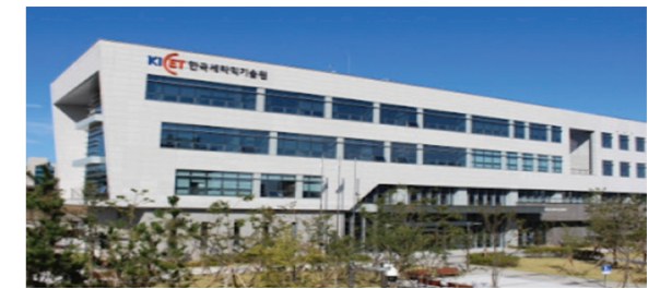
Project Name : Dry Room Cooler Outdoor Fan Repair Client : Korea Institute of Ceramic Engineering & Technology PJT Period : 2021
