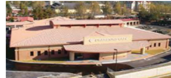
Project Name : COE O-san Church Facility Construction Client : Il-Gwang E&C PJT Period : 2021~Processing
