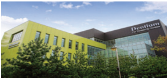
Project Name : Dentium Industrial Center BCR, GMP Construction Client : Heung Deok E&C (Suwon) PJT Period : 2020
