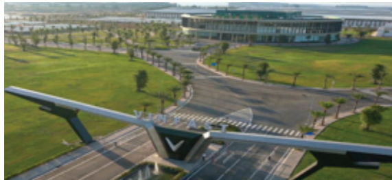
Project Name : VINFAST Dry Room Construction Client : NEWTIMES (Hiphong, Vietnam) PJT Period : 2020~Processing
