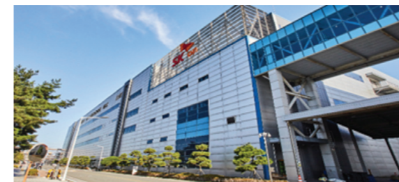
Project Name : SKON Battery #2bd Dry Room Low-Temp Rotor Construction Client : SKON (Seo-San) PJT Period : 2023
