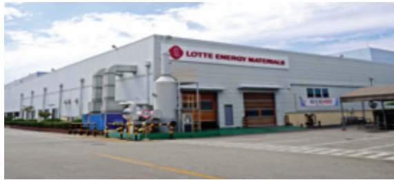
Project Name : All-Solid State Pilot Dry Room Construction Client : Lotte Energy Materials (Ik-San) PJT Period : 2024~Processing
