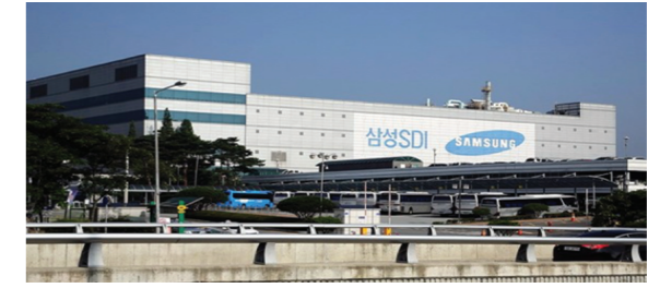
Project Name : Samsung SDI Cheon-An M2bd Rotor Seal Inspection Client : Samsung SDI (Cheon-An) PJT Period : 2023
