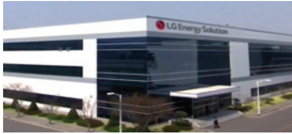
Project Name : LGES DR HVAC Construction Client : LG Energy Solution (Cheong-Ju) PJT Period : 2018~Processing
