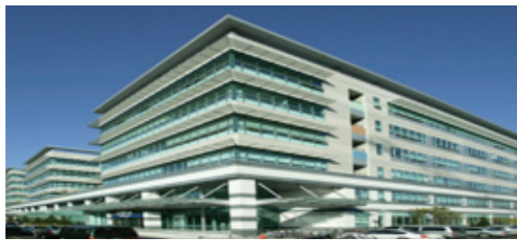
Project Name : SKK LAB Clean Room Design Engineering Client : Sung Kyun Kwan University PJT Period : 2022
