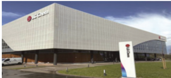
Project Name : O-Chang Small 3rd Bd Electrode Pilot Pipe Construction Client : LG CHEM (Cheong-Ju, O-Chang) PJT Period : 2020
