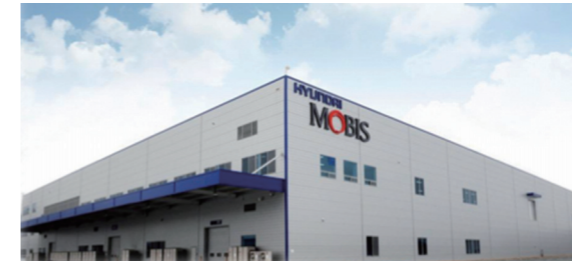
Project Name : CLEAN ROOM SYSTEM Construction Client : Hyundai Mobis (Chung-Ju) PJT Period : 2012
