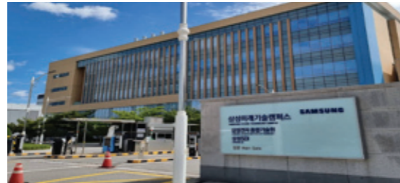
Project Name : Samsung SDI SMRC All-Solid State DR Construction Client : Samsung SDI Future-Tech Campus (Suwon) PJT Period : 2016~Processing
