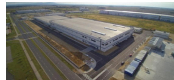
Project Name : LGESWA Coater Heat Exhaust Duct / Hot Oil Pipe Construction Client : LGEnergy Solution (Poland) PJT Period : 2018~2020
