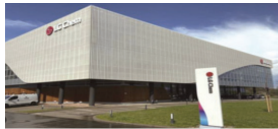
Project Name : LGES Humid HVAC System Design Engineering Client : LG Energy Solution PJT Period : 2023
