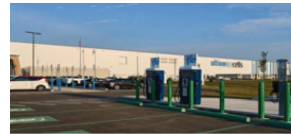
Project Name : Electrode #1 ME BOOTH Construction Client : Ultium Cells(Ohio, U.S.) PJT Period : 2020~2021
