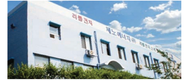
Project Name : Xeno Energy Dry Room Construction Client : Xeno Energy PJT Period : 2017
