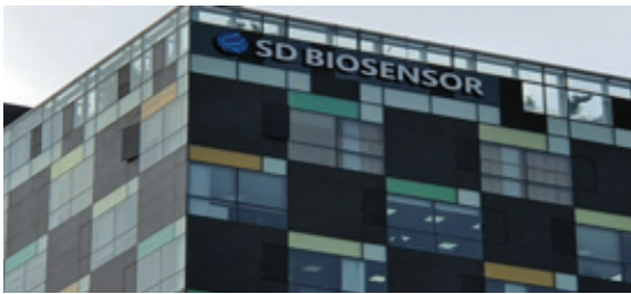
Project Name : SD Biosensor GMP Construction Client : SD Biosensor (Suwon) PJT Period : 2020~Processing
