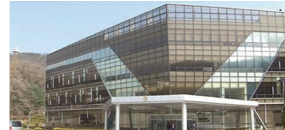
Project Name : ADD Dry Room Construction Client : Agency for Defense Development (Nanjing, China) PJT Period : 2016
