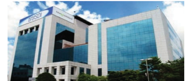
Project Name : ACELine DRY ROOM Construction Client : Samsung SDI (Gi-Heung) PJT Period : 2016
