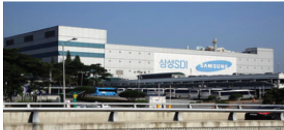
Project Name : Samsung SDI Cheon-An M bd, E bd DR Construction Client : Samsung SDI (Cheon-An, Gi-Heung) PJT Period : 2010~Processing
