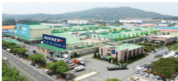
Project Name : Sebang Battery Data Center Precision AC System Construction Client : Sebang Battery PJT Period : 2016~2018
