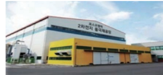
Project Name : Cell Battery Electrode DRY ROOM Construction Client : Posco Chemtech (Se-Jong) PJT Period : 2012 ~ 2015
