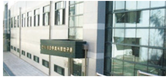
Project Name : Vitzromiltech CLEAN ROOM Construction Client : Vitzromiltech (Pyeong-Taek) PJT Period : 2017
