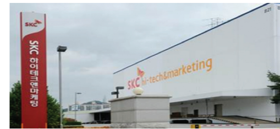
Project Name : Low-Temp. Storage Outdoor Fan Inspection Client : SKC Hi-tech & Marketing PJT Period : 2021
