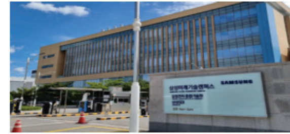
Project Name : [Future-Tech Campus] SDI Dehumidifying HVAC Equipment Maintenance Client : Samsung SDI PJT Period : 2023~Processing
