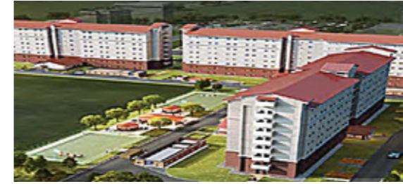
Project Name : FED Enlisted Bachelor Quarters Facility Construction Client : DaeWooE&C, Seilens PJT Period : 2023~Processing
