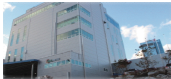
Project Name : Bionote HACCP&GMP HVACFacilityConstruction Client : Bionote (Hwa-Seong) PJT Period : 2020~Processing
