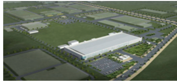
Project Name : LGCN Dry Room Construction Client : LGEnergy Solution (Bingang, China) PJT Period : 2019~Processing
