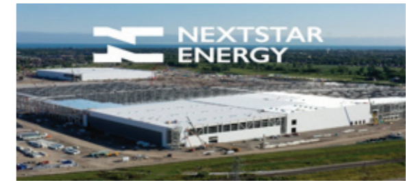
Project Name : Electrode #1~6 Heat Exhaust Duct & Hot Oil Pipe Construction Client : Nextstar Energy(Windsor, Canada) PJT Period : 2022~Processing
