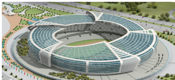
Project Name : Stadium Precision AC System Construction Client : Securo (Baku, Azerbaijan) PJT Period : 2012
