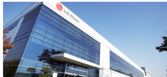
Project Name : LG CHEM Low-Temp Storage, Precision AC System Facility Construction Client : LG CHEM (Cheong-Ju) PJT Period : 2013 ~ 2016
