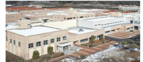
Project Name : FED Humphrey Prison Facility Construction Client : Woo Seok E&C PJT Period : 2021~Processing
