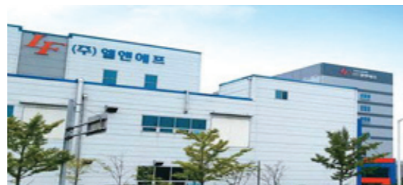
Project Name : 3rd Factory Battery DR Construction Client : L&F (Dae-gu) PJT Period : 2023~Processing
