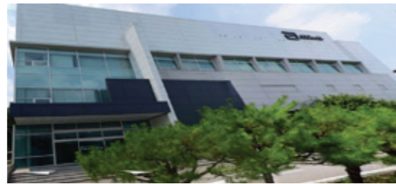
Project Name : Abbott GMP Construction Client : Abbott (Yong-In) PJT Period : 2012~Processing
